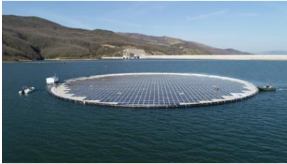
Fig. 1. An existing Floating photovoltaic unit on the water reservoir of a hydro power plant
